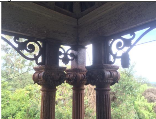
Figure 62: First Floor balcony's corner columns
